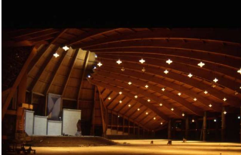
Glued laminated indoor structure at the Mary Queen of the Apostles Basilica in Yaoundé - Cameroon (© Jean Uhalde, UBC).
